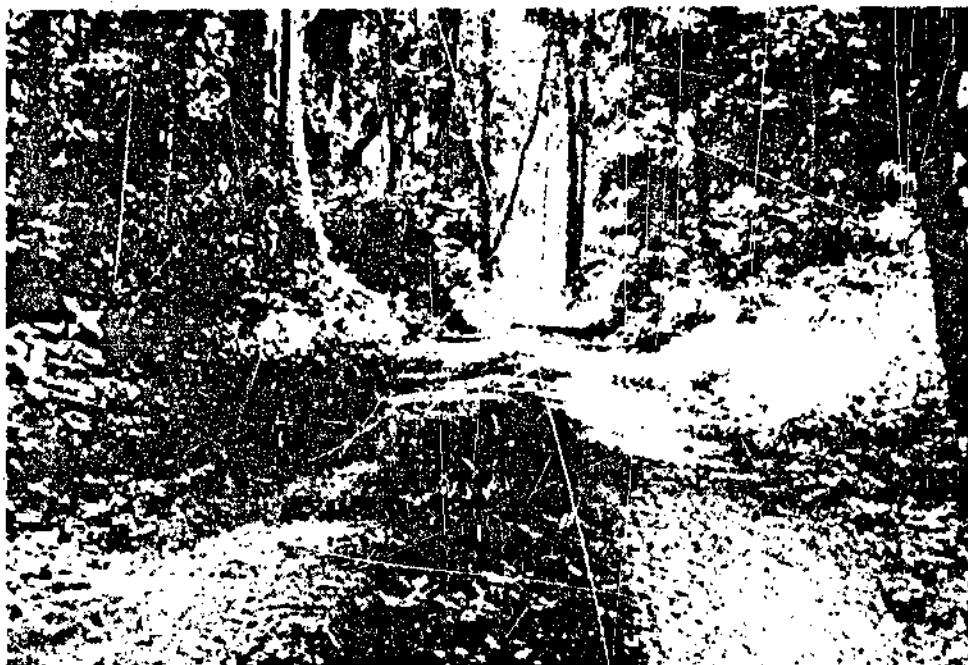
Figure 94.-Forest road on heavy, red volcanic clay as it appeared after 2 years of use by light vehicles during all seasons, and heavy trucks in dry season. Between Sala Dar and Sopheas, Cambodia.
